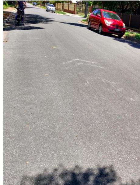
These pictures show the value of thermoplastic line marking when it comes to bike logos. The photo on the left is of the Frome Bikeway as it leads into Halifax Street. The closest logo was painted normally. The furthest is thermoplastic.
