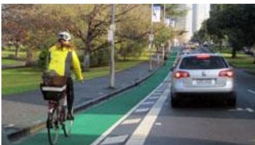
As parking provides clearance to moving traffic, only a painted buffer to car parking is required. It is desirable but not entirely necessary that the bike lane be coloured green. If it is not, then we recommended a 'strongly' painted buffer as shown in the Melbourne example, featuring solar LED cateyes on the carparking edge to emphasise its presence.
